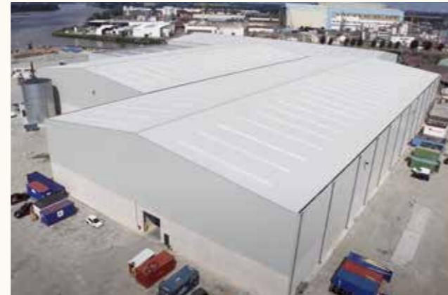
1Plant's strategic location allows for more efficient transportation.
